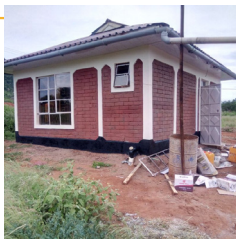
Hydraform Soil Interlocking Block (9by x 8by 115mm)
